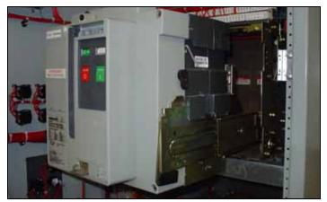
Figure 14. Drawout Mechanism (Closed Transition Shown)
